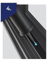
Prior to fixing the frame, seal the holes in the bottom of the frame to prevent water ingress.
