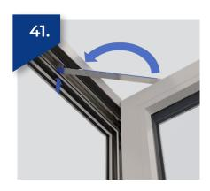
Open the sash to desired maximum opening angle, hold or wedge to keep it in place, and then position the restrictor arm to determine frame bracket location.
