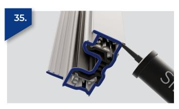
Run a continuous bead of silicone sealant around the joint between the end-milled frame and the threshold.
