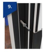
Remove side cover trim before fixing through the centre of the thermal break as shown.
