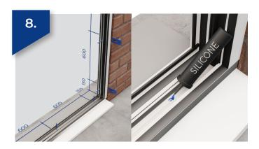
Drill and fix the frame at 150mm from each end, and no more than 600mm between centres. Fit packers at the same locations. Ensuring the head of screws are below the bottom of the track, to prevent the rollers colliding. Sealing the bottom fixing locations to prevent water ingress. Please note points 9 and 10 for side fixings.
